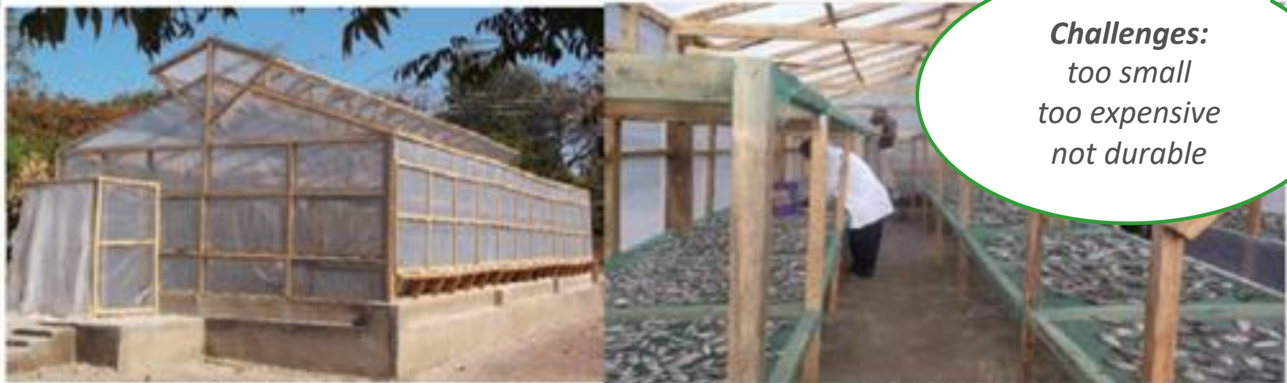
Figure 1: Picture of outside and inside view the design of the solar tent dryer that was adopted
